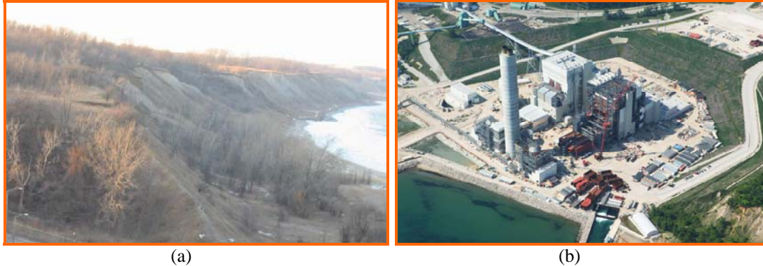
Figure 1. Construction site along the shoreline of Lake Michigan: (a) before excavation; (b) during construction.
